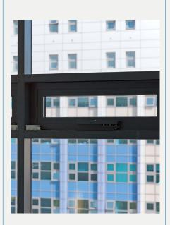
SE Controls were specified on the project as they were recommended by the window specialist, the SECO 20 Chain Actuator provided a low power drain on the BMS system as compared to other actuators currently available. By choosing low amperage actuators, cost savings can be made both in the fixed hardware required for control and save energy requirements over time.
